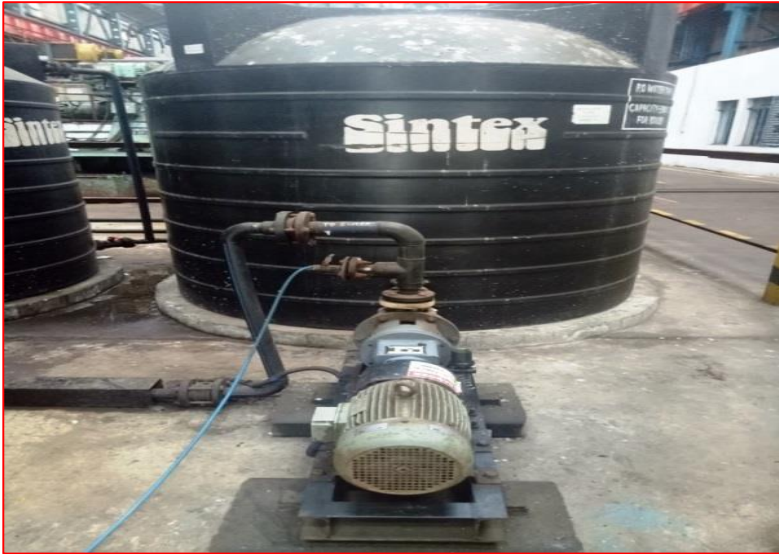
Reduction of water consumption by using self-cooling pumps
