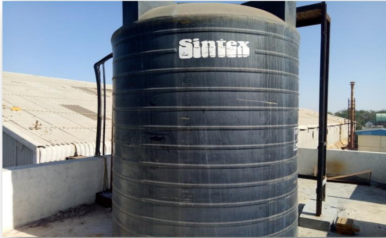
Overhead Storage tank for RO Rejected water
