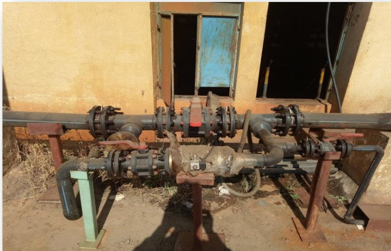
Auto Control Valve Station
